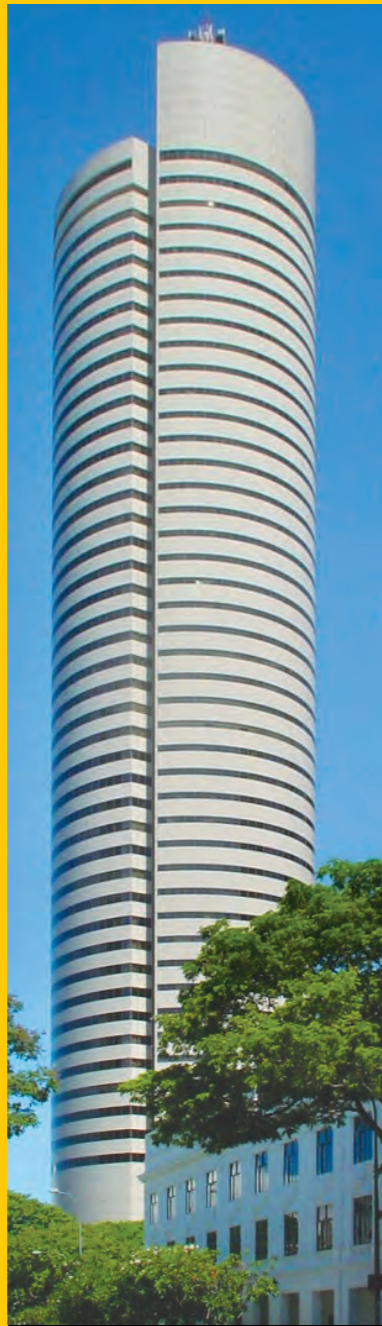
AXA Tower at 8 Shenton Way
