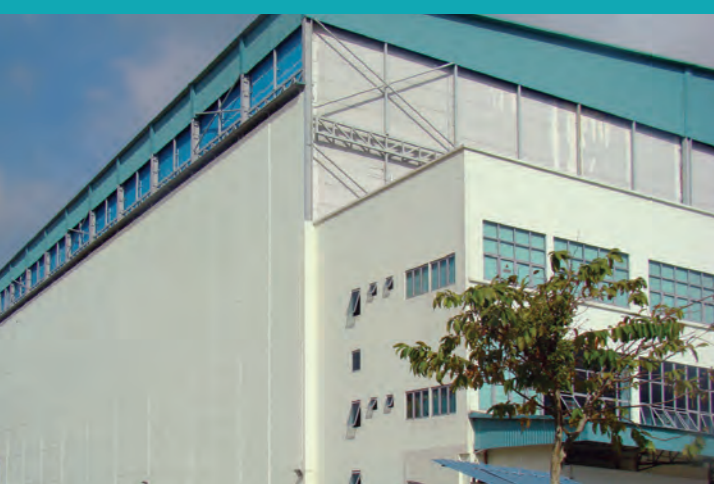
Mandai Link Logistics' Warehouses-Cold Storage at Mandai Link
