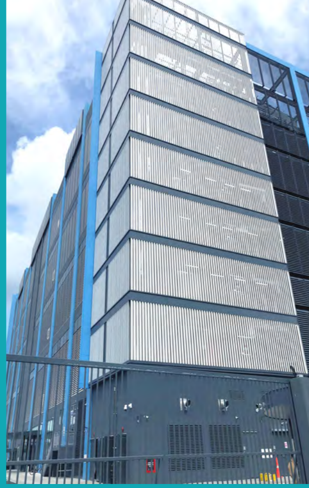
Data Center at Loyang Drive
