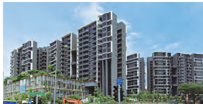
Grandeur Park Residences Condominium
