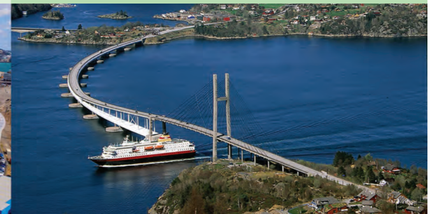
The Nordhordland Floating Bridge
