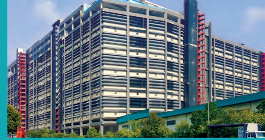
6 Storey Warehouse at 47 Jln Buroh
