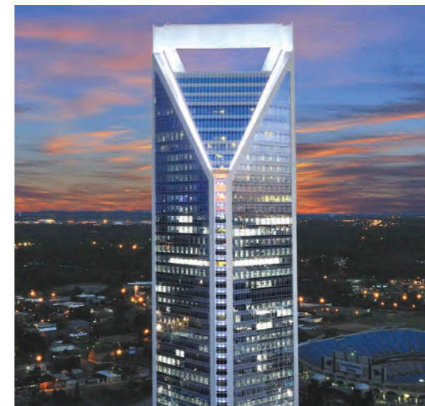
Duke Energy Centre (USA)
