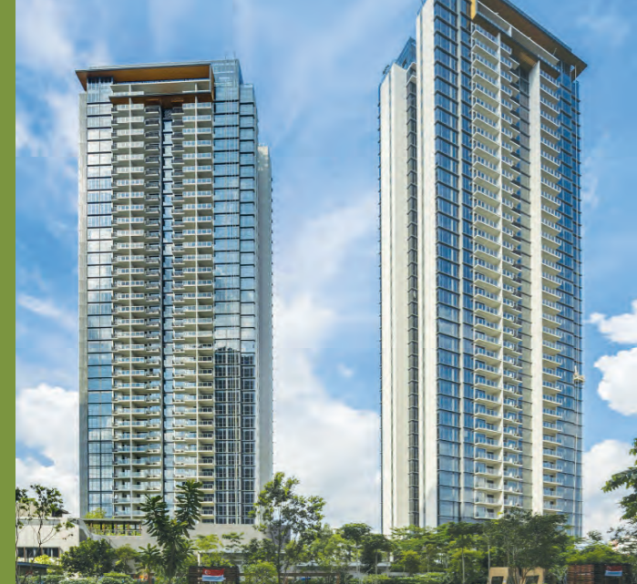
Twin VEW Condominium
