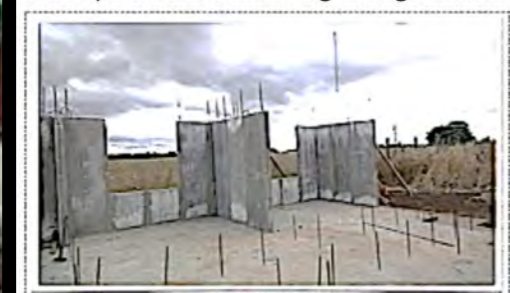
Wire Reinforced Panel Joints Solid, Strong, Full Contact Minimize Seismic Impact
