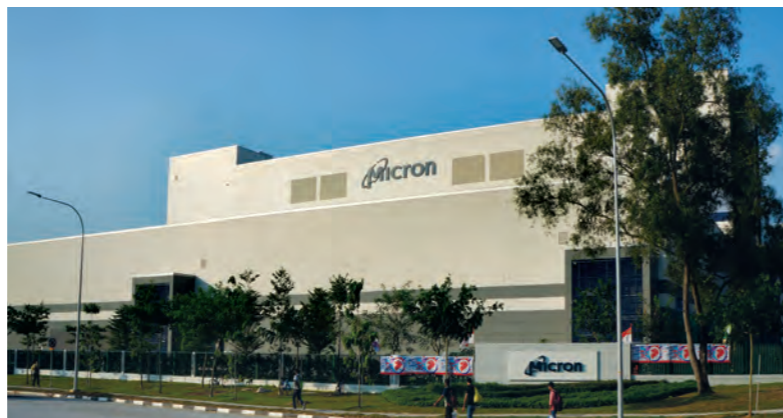
Micron 300mm NAND Facility at 1 North Coast Drive
