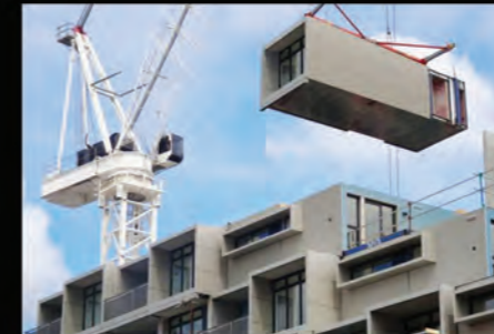
PPVC & PBU Precast
