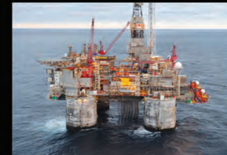
Insulation of Pipeline in Oilfield
