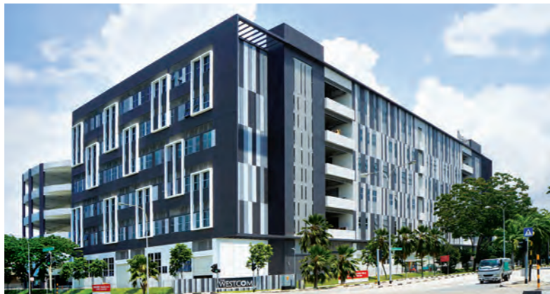
THE WESTCOM at 1 Tuas South Avenue 6
