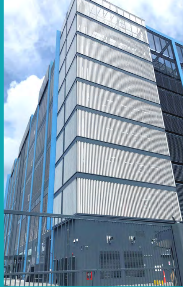
Data Center at Loyang Drive
