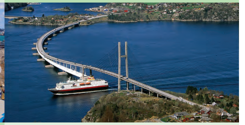
The Nordhordland Floating Bridge
