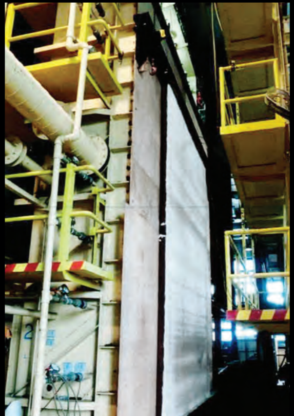
AIR TIGHTNESS TEST Air Transmission = 0% TUV Certified
