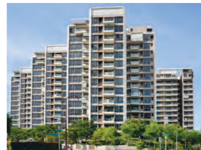
KOVAN REGENCY Condominium
