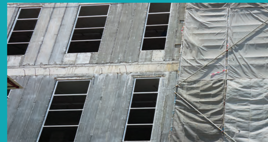
Using panel 5.2m height for external wall and window opening
