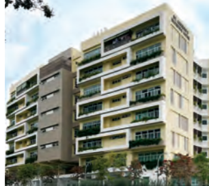
St. Andrew's Nursing Home at Jalan Penjara
