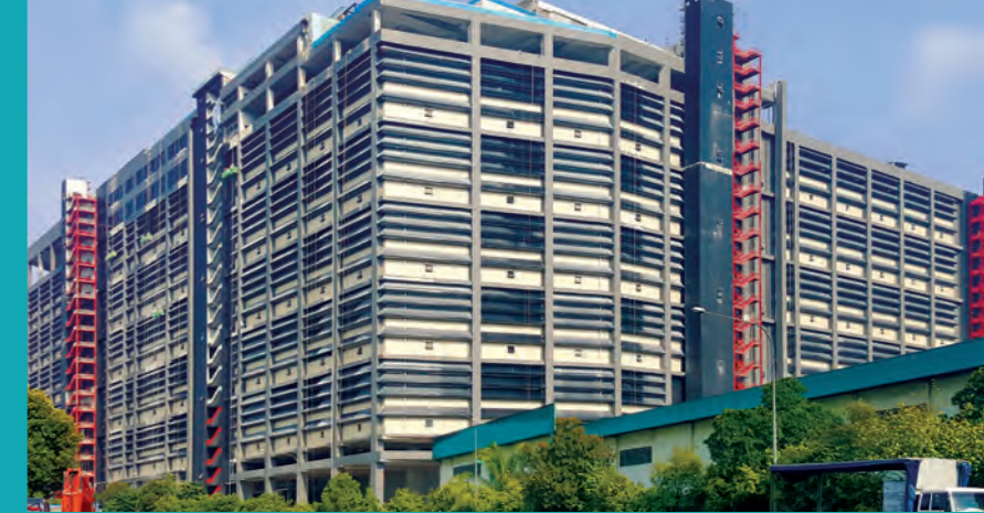
6 Storey Warehouse at 47 Jln Buroh
