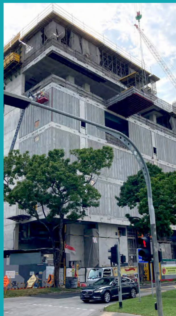
STTelemedia Global Data Centres at 51 Defu Lane 10
