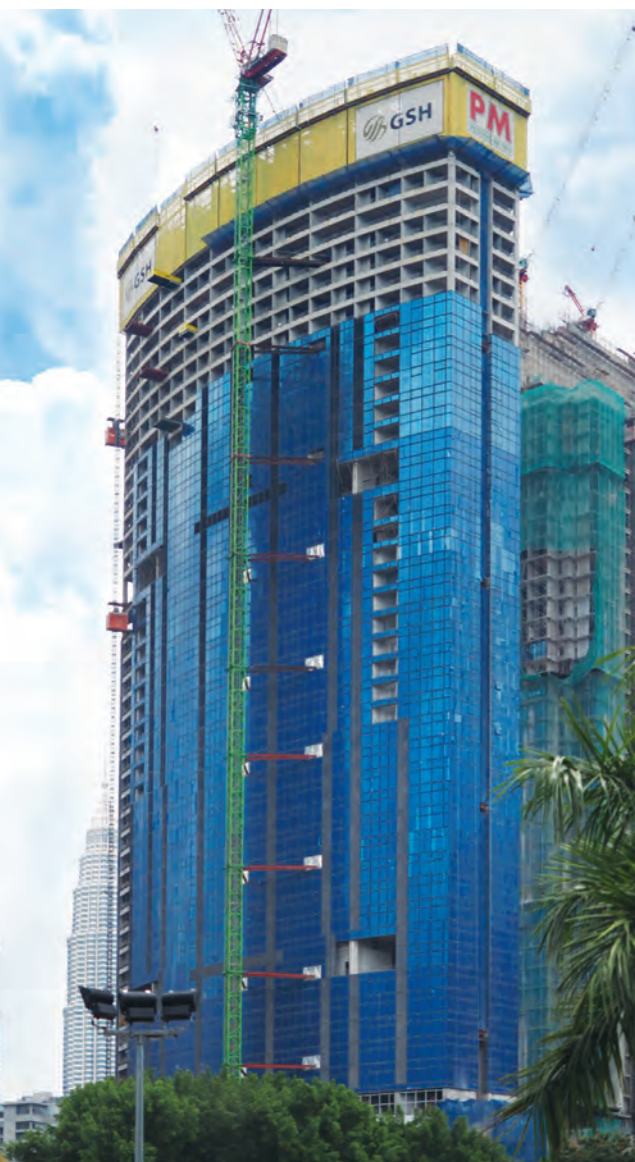
EATON RESIDENCES at Kuala Lumpur, Malaysia
