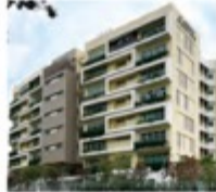
St. Andrew's Nursing Home at Jalan Penjara
