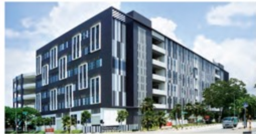
THE WESTCOM at 1 Tuas South Avenue 6
