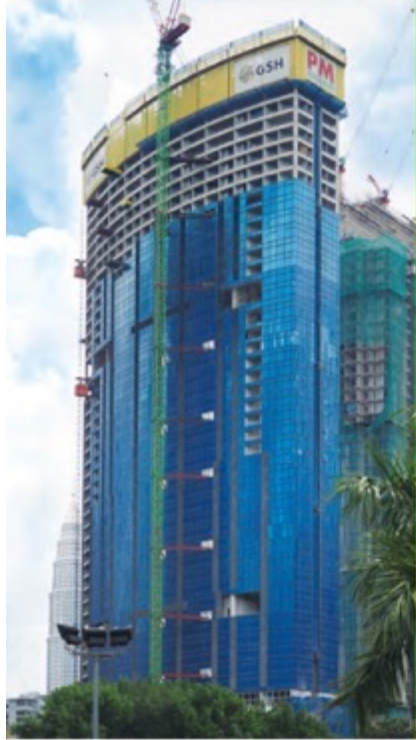
EATON RESIDENCES at Kuala Lumpur, Malaysia
