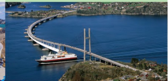
The Nordhordland Floating Bridge
