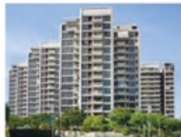
KOVAN REGENCY Condominium
