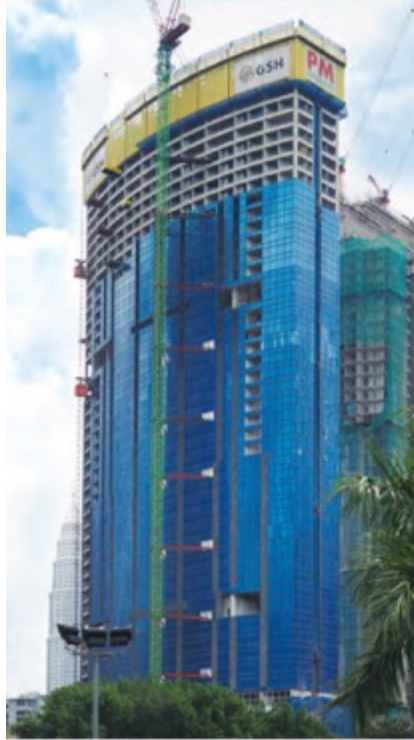
EATON RESIDENCES at Kuala Lumpur, Malaysia
