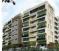
St. Andrew's Nursing Home at Jalan Penjara
