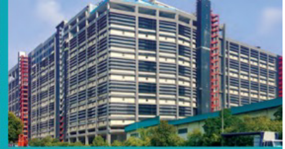
6 Storey Warehouse at 47 Jln Buroh
