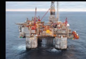
Insulation of Pipeline in Oilfield
