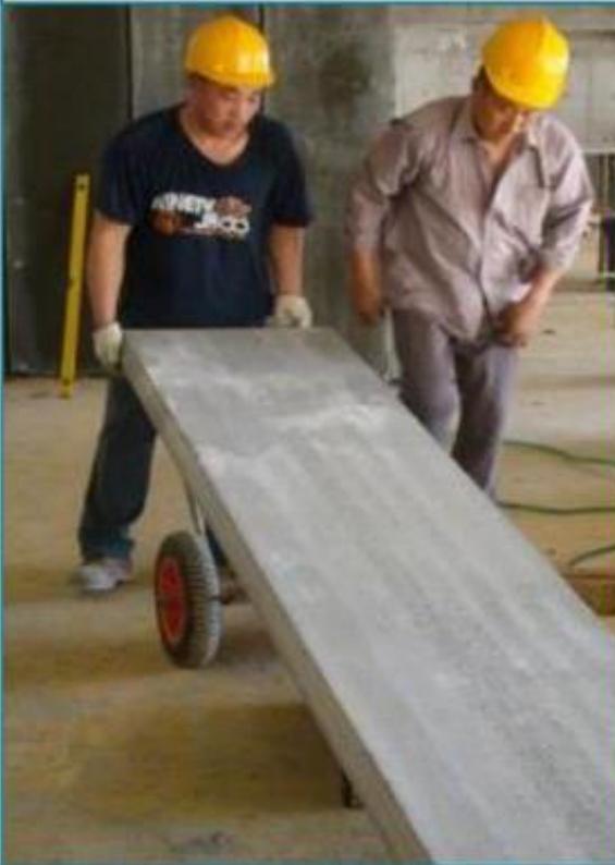
Use Trolley to Move Panel
