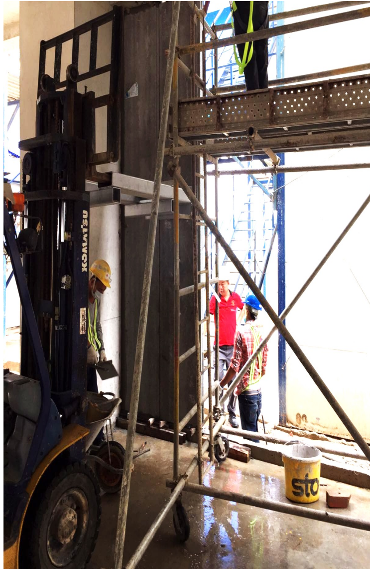
Using Forklift and Lorry Crane for Lifting and Installation
