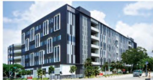
THE WESTCOM at 1 Tuas South Avenue 6
