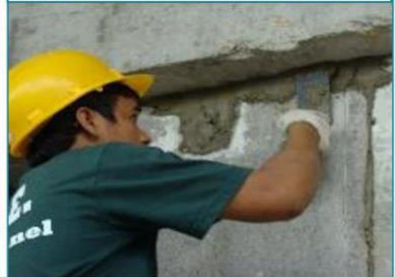
Apply JOE JOINT BONDING Adhesive
