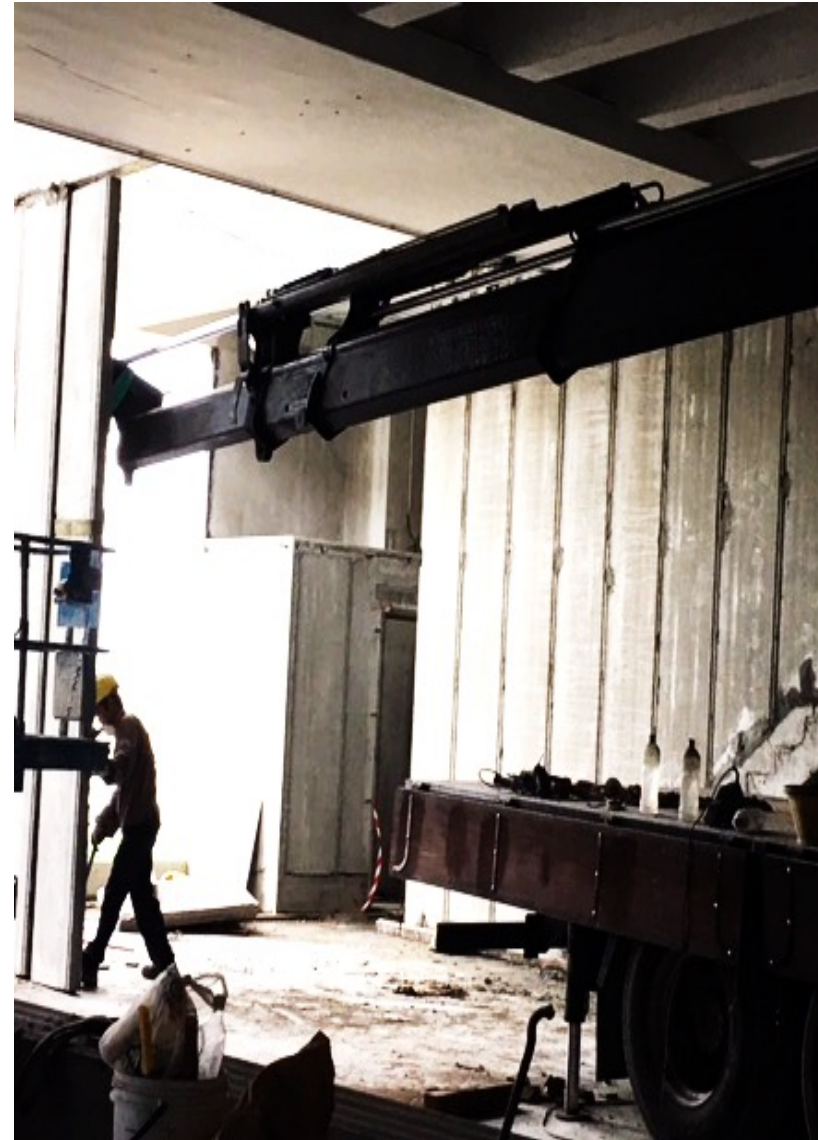
Using Forklift and Lorry Crane for Lifting and Installation
