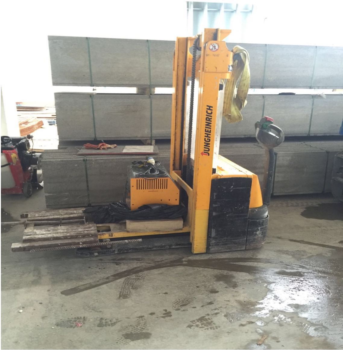
Using Electric Stacker for Lifting and Installation
