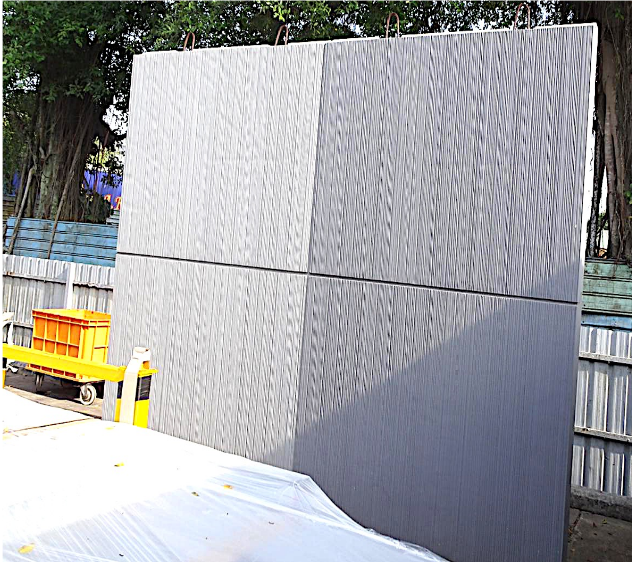
Precast Facade using Form-liner molding – Wavy & occupy crantage hours
