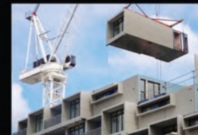
PPVC & PBU Precast
