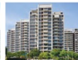
KOVAN REGENCY Condominium
