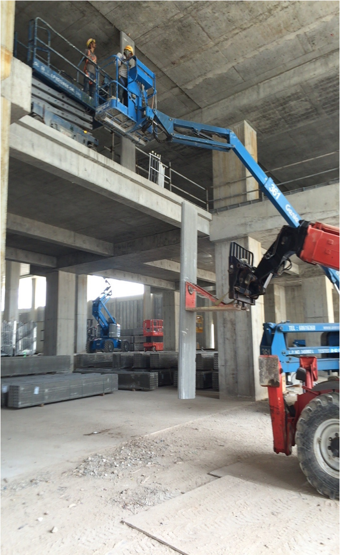
Using Forklift and Scissor Lift for Lifting and Installation
