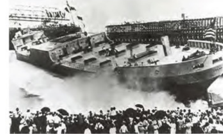
Launching of Lightweight Concrete Ship U.S.S. SELMA in 1919 Year 1919 : 26.7 MPa Year 1980 : 55.2 MPa
