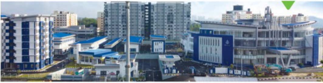
Additional Buildings In Johor State CIDB Complex at Jalan Tampoi, Johor Bahru, Malaysia
