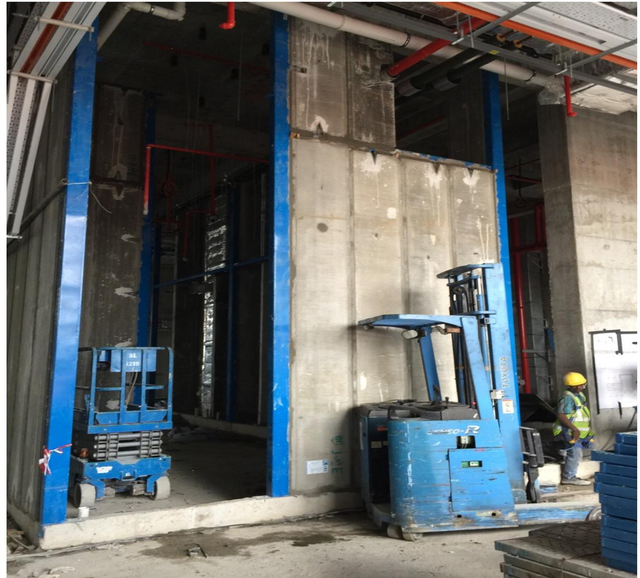
Using Electric Stacker for Lifting and Installation
