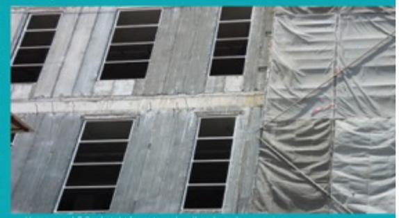
Using panel 5.2m height for external wall and window opening
